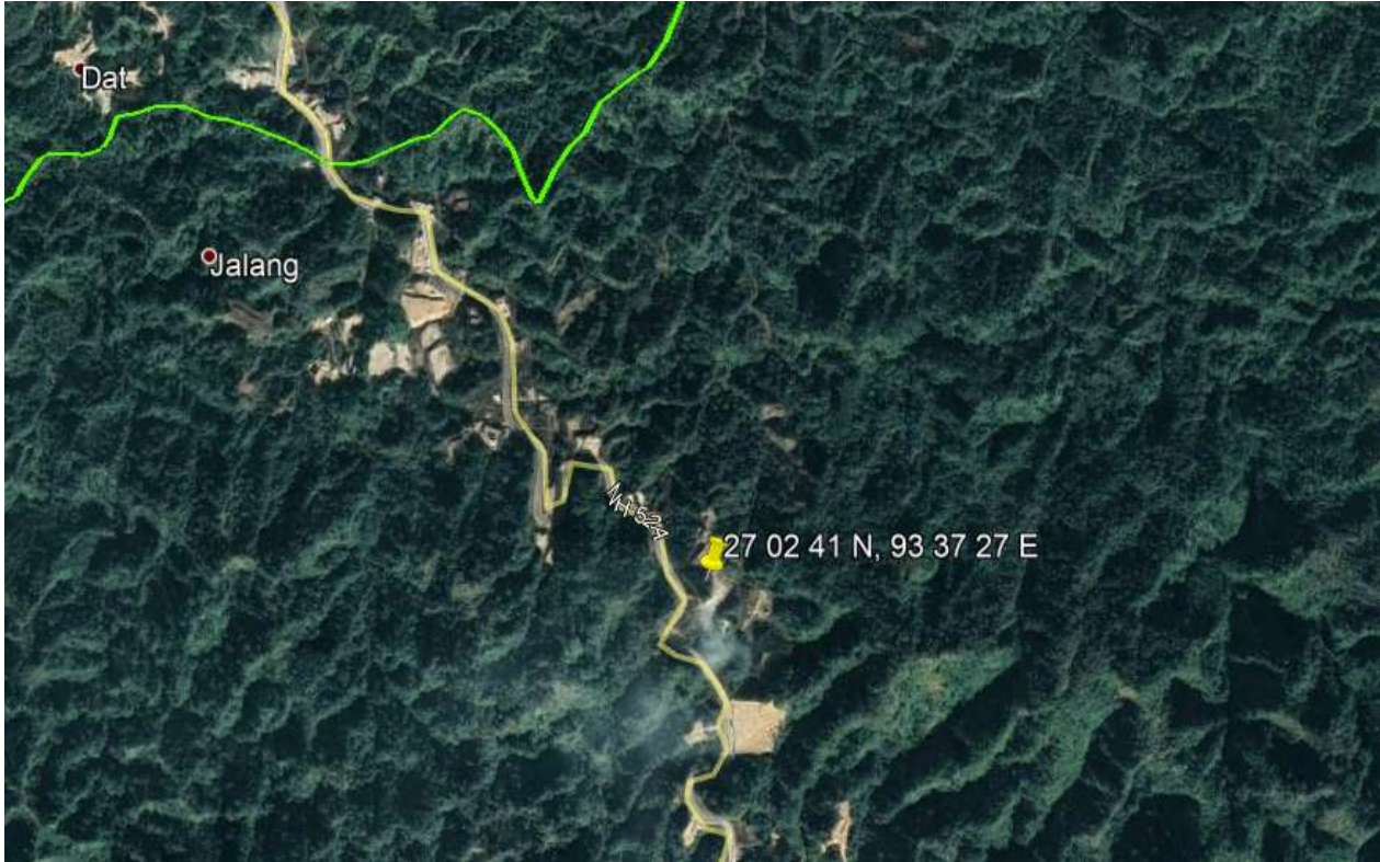
Picture 10: Municipal Solid Waste (MSW) Plant Chimpu, Itanagar
