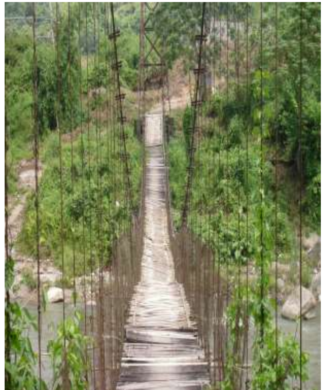
Picture 3: Temporary Link across River
