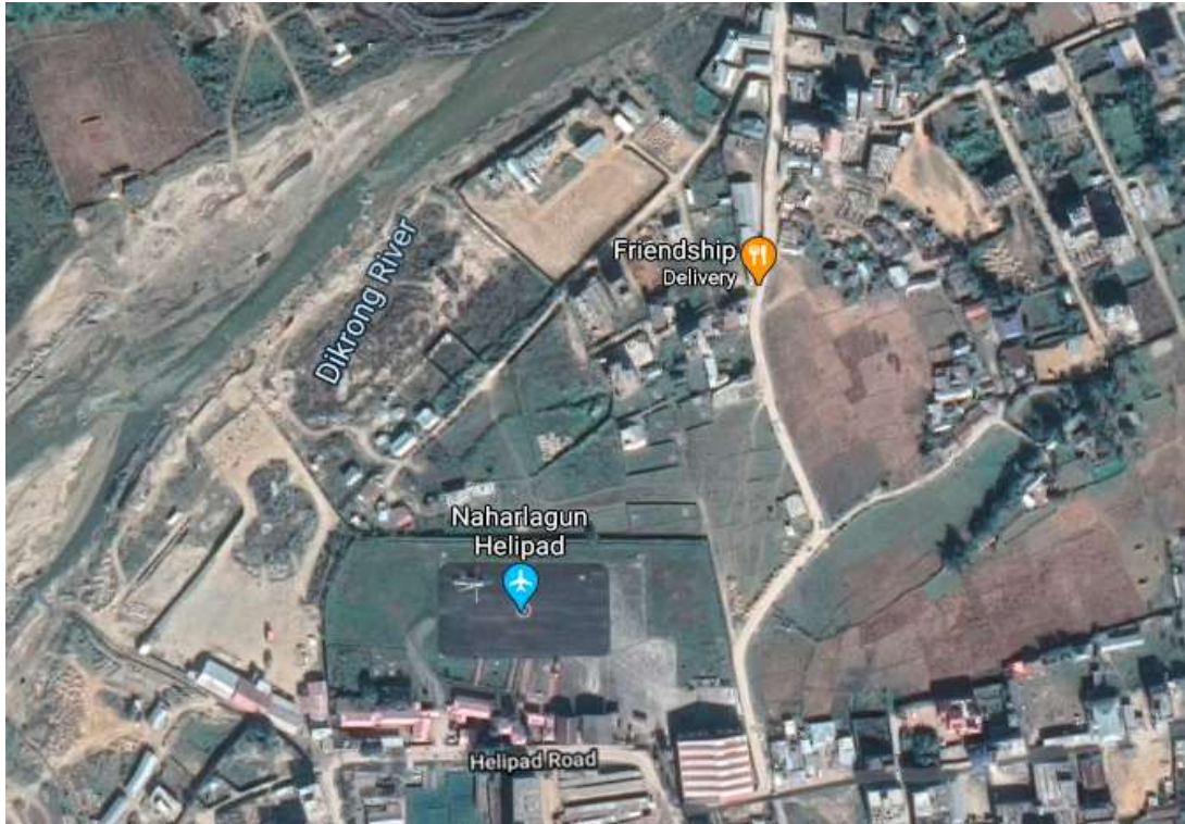
Picture 15: Proposed Sewerage Treatment plant in Naharlagun
