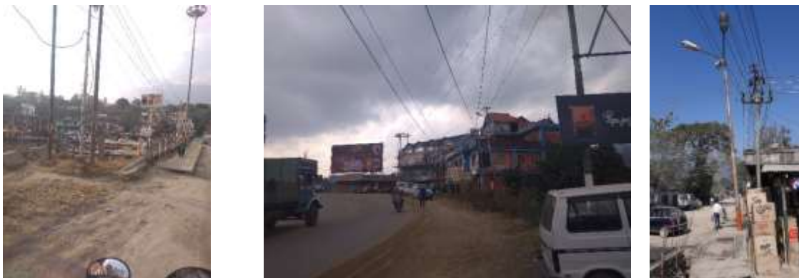
Picture 12: Power lines Condition in ICR
